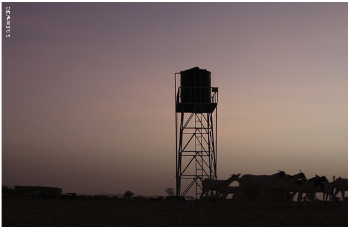
Mali, 2021: Water tower installed by the ICRC to support villagers affected by combined effects of conflict and climate change.
