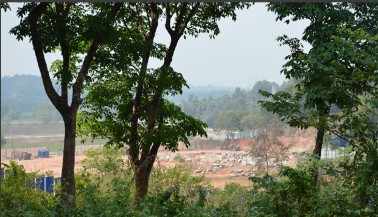
Resettled families displaced by the Smart City in Kochi, Kerala now look over a construction site on their former land. Local resettlement has enabled residents to maintain community ties and maintain proximity to schools and healthcare facilities, however the loss of jobs dependent on agricultural land have not been compensated. See case study on page 30. Credit: IDMC, March 2016
