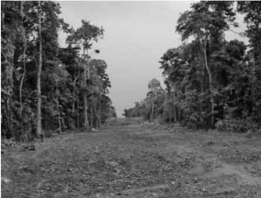
View of the pipeline near Kribi, Cameroon. A swath of forest 100 feet (30 meters) wide was cleared for the pipeline route for 665 miles (1,070 kilometers), from oil fields in Chad to the Atlantic Ocean port in Kribi. The pipeline is buried 3 feet (1 meter) underground.
